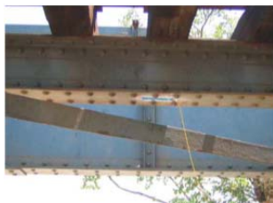
(a) The instrumented bridge
