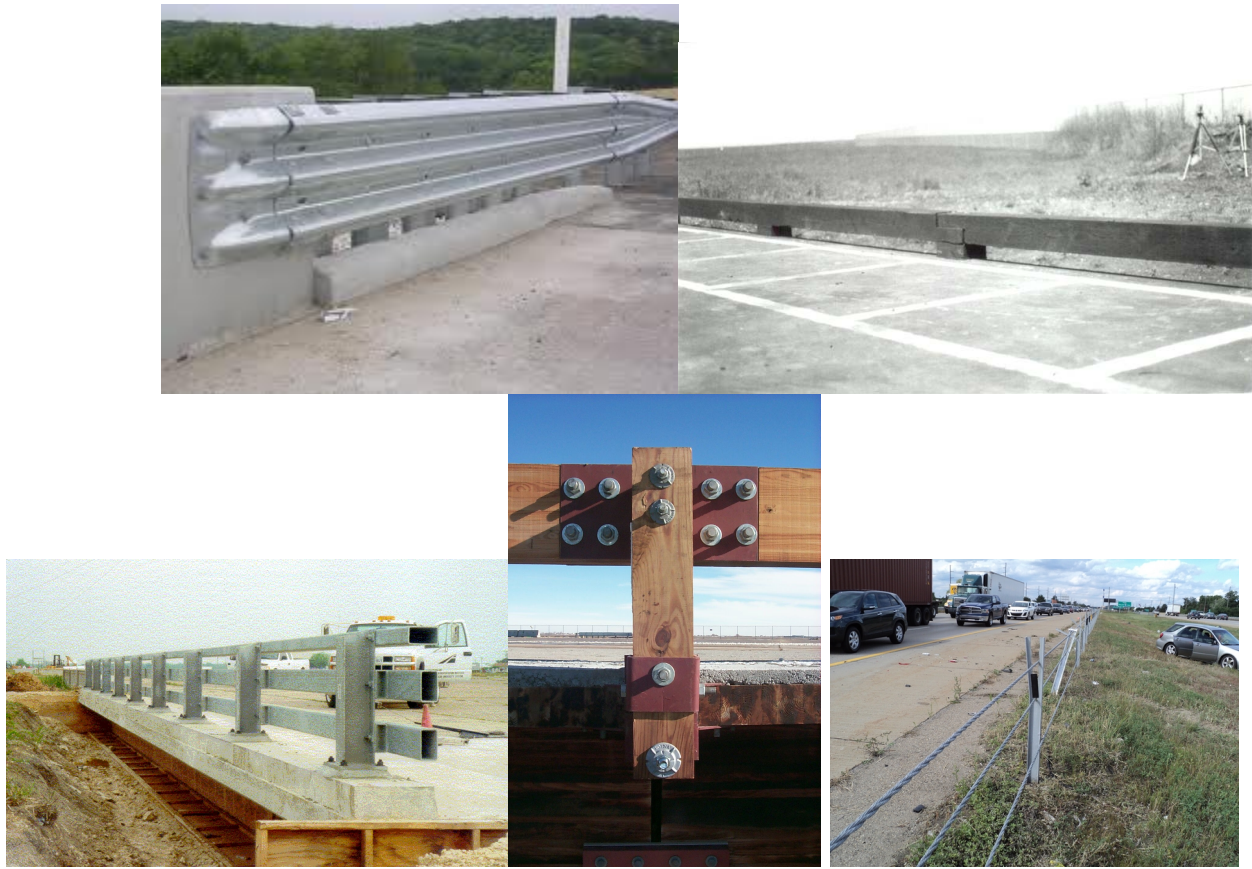
Figure 1. Clockwise from upper left: (a) The standard three-beam guardrail, (b) typical curb-type timber bridge rail, (c) cable shoulder barriers after an accident, (d) connection details for a solid wood post and glulam railing, and (e) steel tubing rails with I-section posts.
